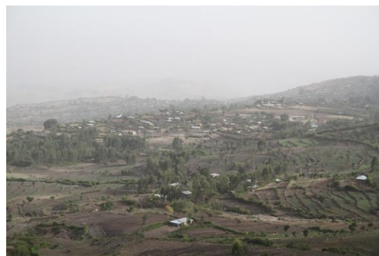
Recently installed soil conservation terraces on Choke Mountain. EPS researchers are studying the efficacy of these structures in a changing climate.
